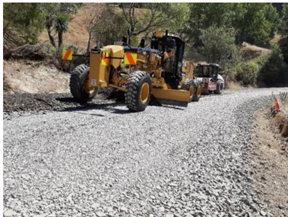
Pavement Work – Route 52
