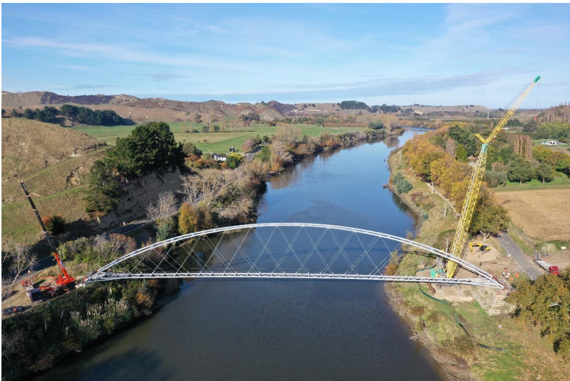
Photo: Launching of the Upokongaro Cycle bridge across the Whanganui River
