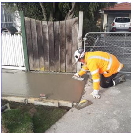
Footpath Maintenance works - Woodville
