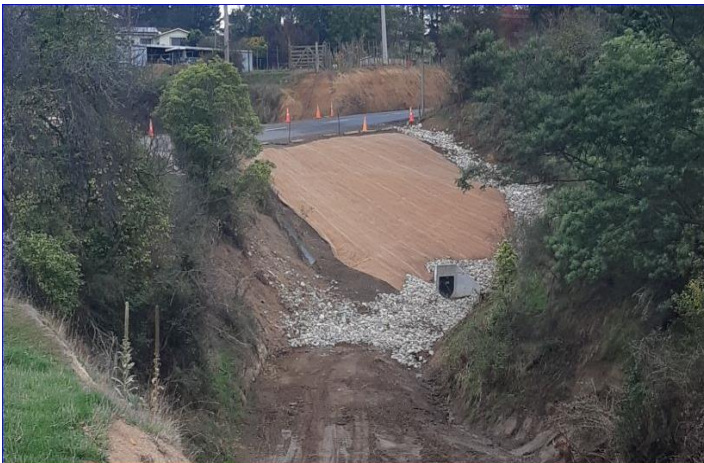
Norsewood / Ormondville Road, Pipe Jacking Project nearing completion
